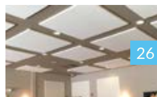
SOUND MANAGEMENT Masking, Dampening and Blocking
